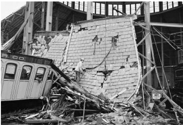
Figure 1(b) Roundhouse Postcollapse (Courtesy of The B&O Railroad Museum)
